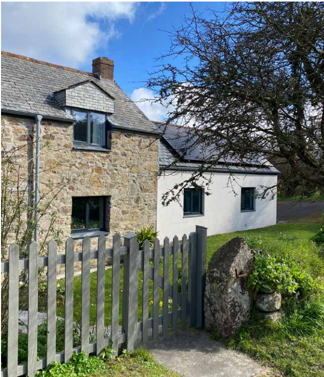
Figure 12 Typical residential building in Trevail. This barn conversion (left) with modern extension (right) has a sympathetic architectural material palette of a white render and local rubble stonework facades with a grey tiled roof.
