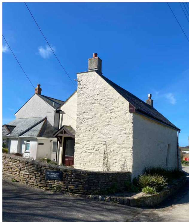
Figure 16 Historic white rendered rubble and cob building with a unique building form, which is situated in a prominent location along the main street of the hamlet.
