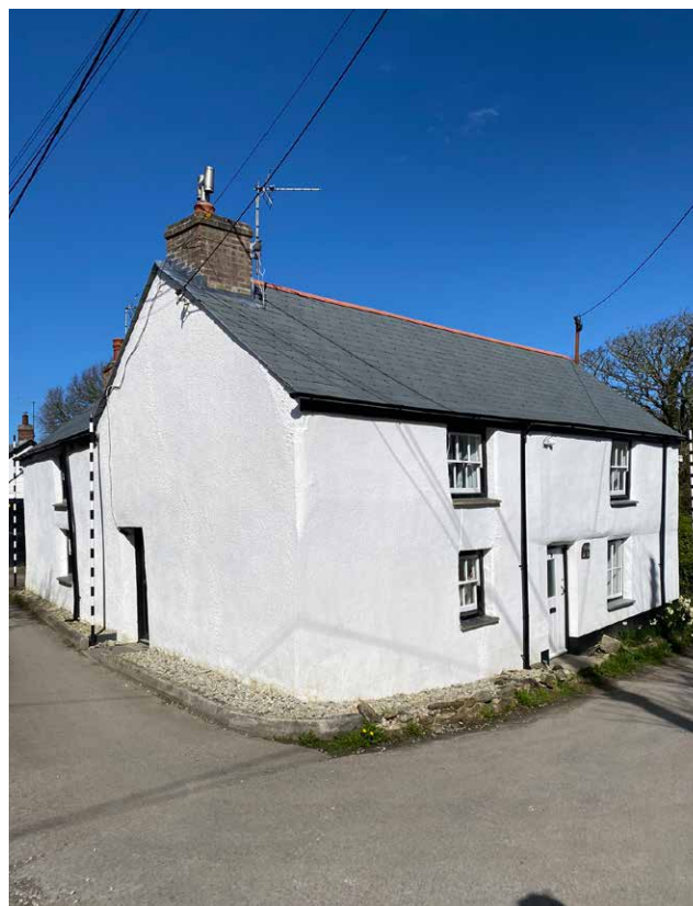
Figure 8 Typical residential building in TreSean. The white render facade with a grey tiled roof is the prevailing character. White sash windows and doors, and simple brick chimneys are also prevailing architectural features.
